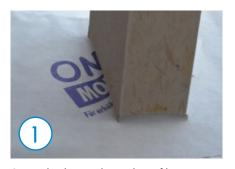
Cut out the chimney duct at the roof laying membrane.
