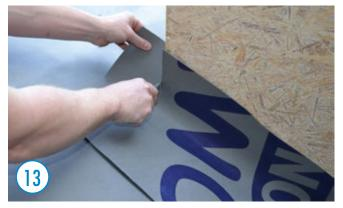
In the upper chimney area, also allow for a lateral overhang of approx. 10 cm and cut it off along the upper corner of the chimney.
