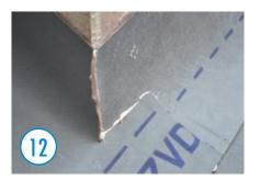
Seal all connections and overlaps in the lower area with the OMEGA QUILLI adhesive sealant.
