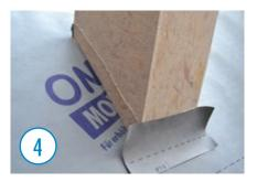
Also apply the OMEGA QUILLI sealant to the side of the chimney.
