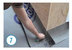
Cut along the front edge of the chimney. seal.
