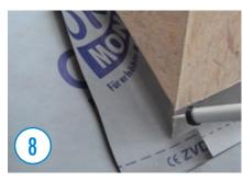
Corner area with the OMEGA QUILLI adhesive sealant
