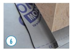
Lateral elevation at least 15 cm up the chimney, but at least 2 cm over the upper edge of the counter battens
