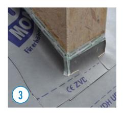
The upper connection area can also be sealed around the chimney with the AIRSTOP ULTRA adhesive tape.
