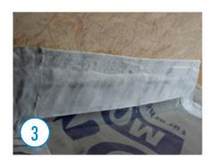
The lateral connection strips on the chimney can also be executed with the OMEGA PLASTO tape. If necessary, apply primer beforehand.
