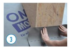
Run the lower connecting strip 15 cm up the chimney (but at least 2 cm above the upper edge of the counter batten).
