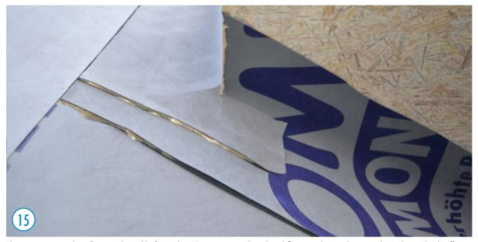
Above penetrations and installations with a width of more than 50 cm, transverse channels or deflection angles must be arranged on a slope and with sufficient lateral overhang.
