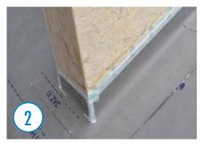
In addition, the upper connection area can be sealed with AIRSTOP FLEX adhesive tape. If necessary, apply primer beforehand.
