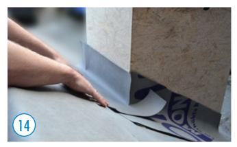
Also run the upper connecting strip at least 15 cm up the chimney - but at least 2 cm above the upper edge of the counter battens.
