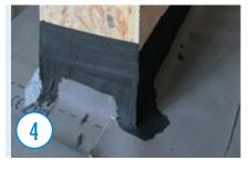
Optionally, the areas covered with AIRSTOP FLEX adhesive tape can be coated with OMEGA PoBit sealing paste.
