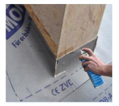
If the upper connection area is sealed with an AIRSTOP adhesive tape, pre-priming (e.g. with the UNI SPRAY spray primer) is recommended.
