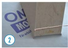
Starting in the lower area, apply the OMEGA QUILLI sealing compound to the chimney.
