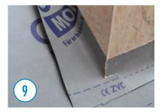
Tape the lateral connecting membrane on both sides of the roofing membrane with the OMEGA QUILLI adhesive sealant so that it is rainproof.
